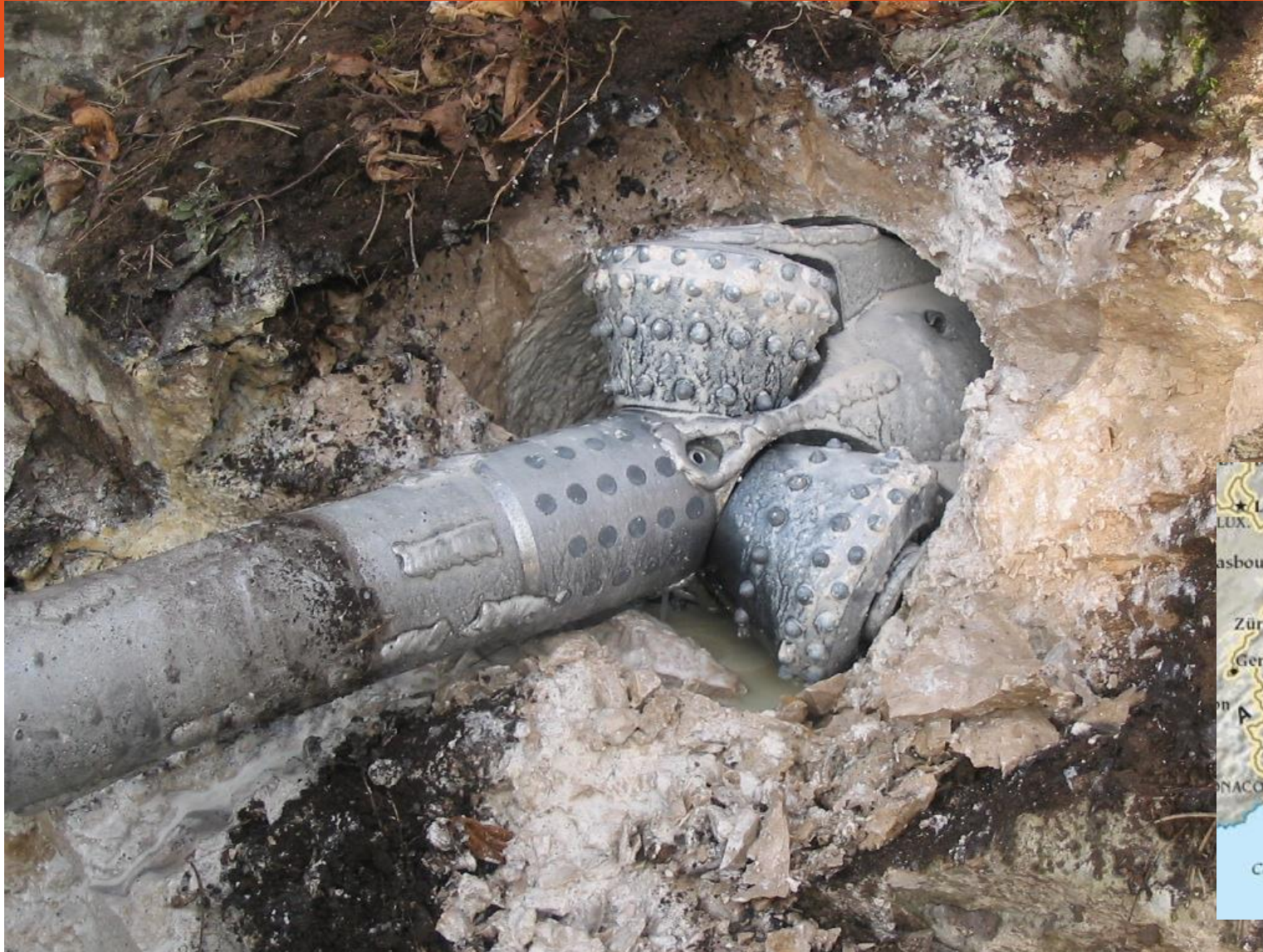
HDD Hole opener in operation in Postojna
